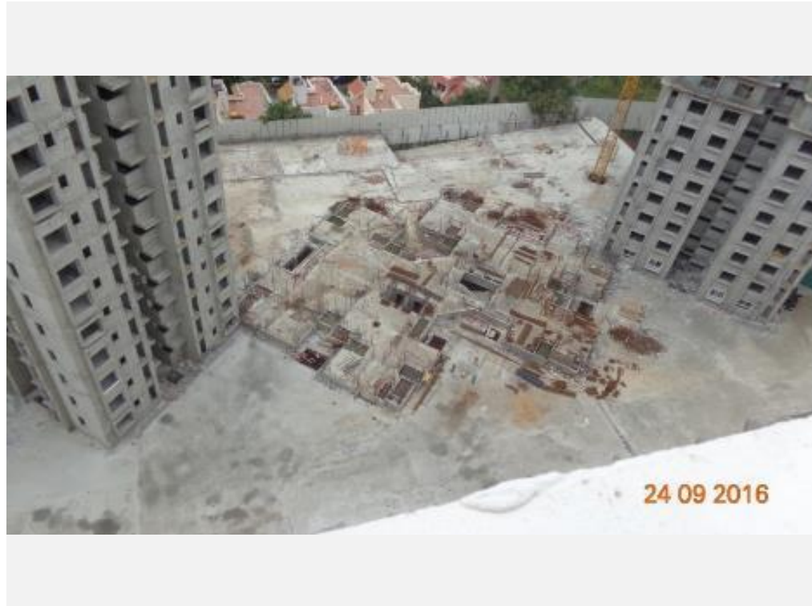
TOWER J Level 2 Work In Progress
